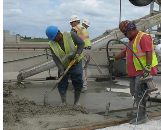
(b) Spreading and initial vibration
