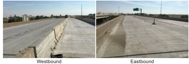
Finished overlays before opening to traffic
