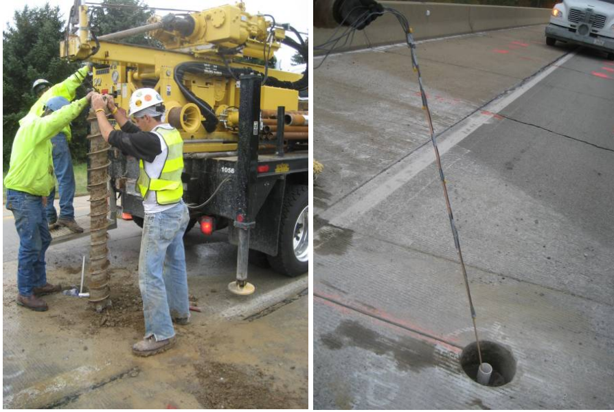
Figure 10. I-button installation
