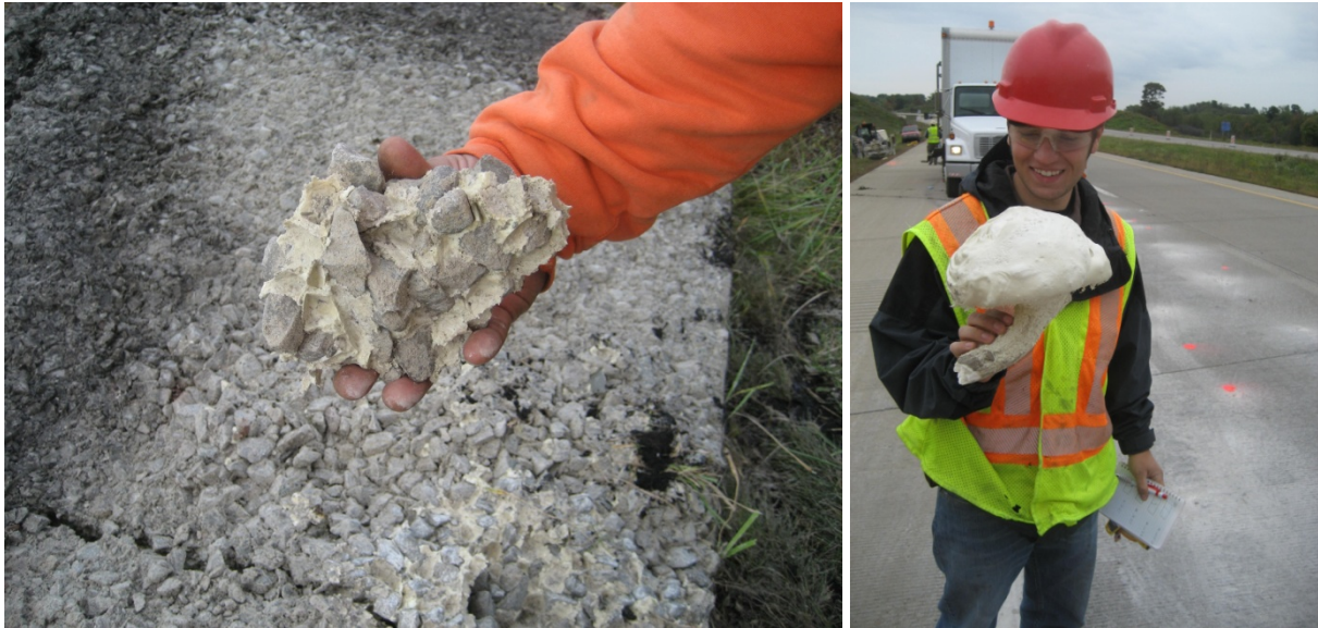
Figure 18. Foam+aggregate mixture (left) and HDP foam ejected through a hole drilled in the pavement (right)
