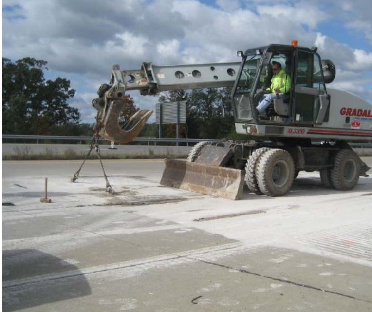
Figure 32. TS1: Crane lifting the PCC surface layer of a patch area
