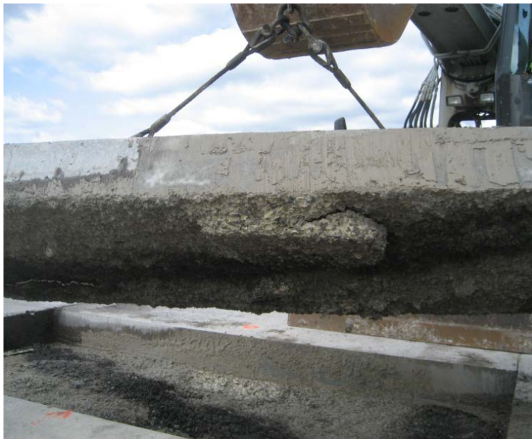
Figure 33. TS1: Bottom of the PCC surface layer in the patch area with treated subbase layer
