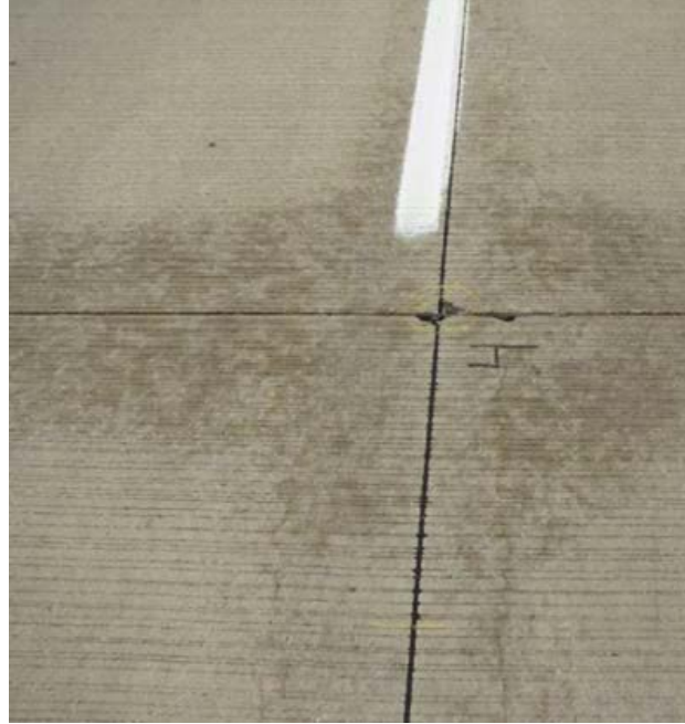
Figure 1. Typical shadowing with trapped water and micro-cracks (Taylor 2011)
