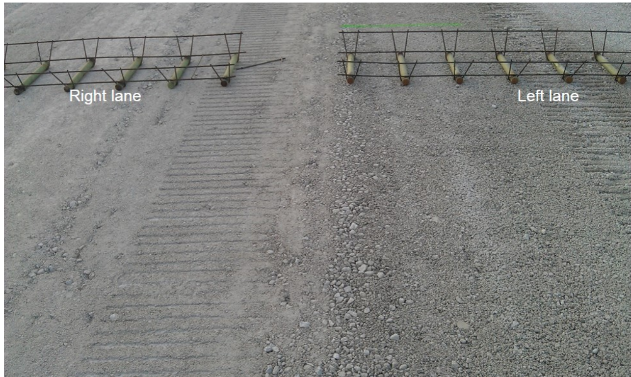
Figure 94. RPCC modified subbase layer surface
