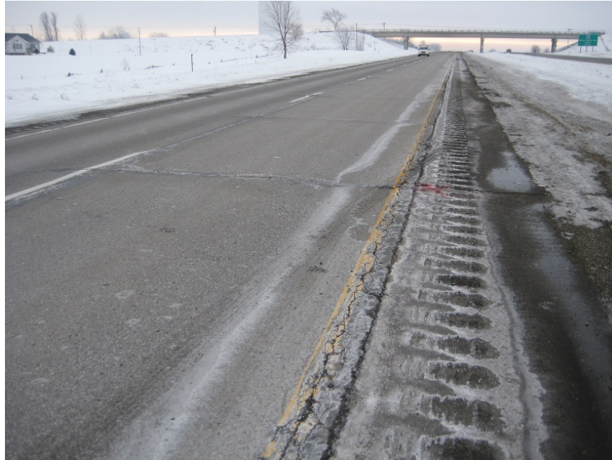
Figure 70. The existing pavement on US 30 EB showing severe surface distresses
