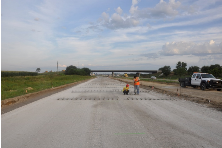
Figure 88. Field testing on finished RPCC modified subbase layer (June 8, 2011)
