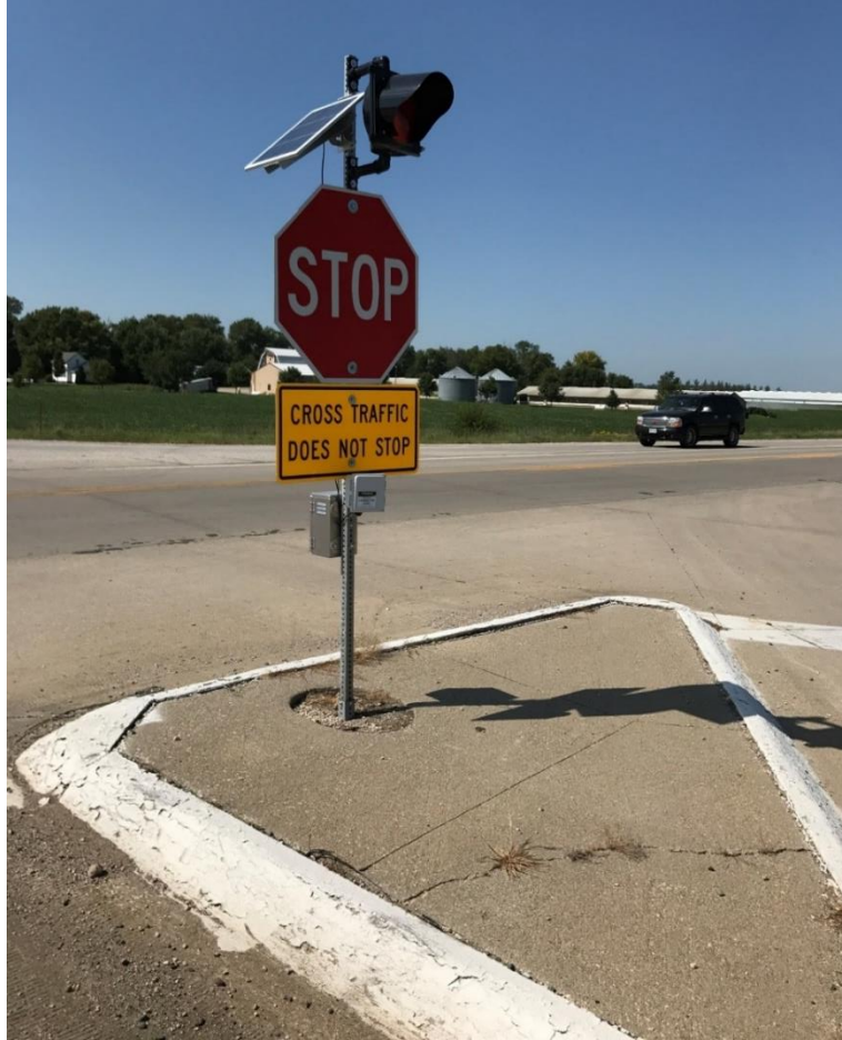
Figure 3-1. Flashing beacon installation
