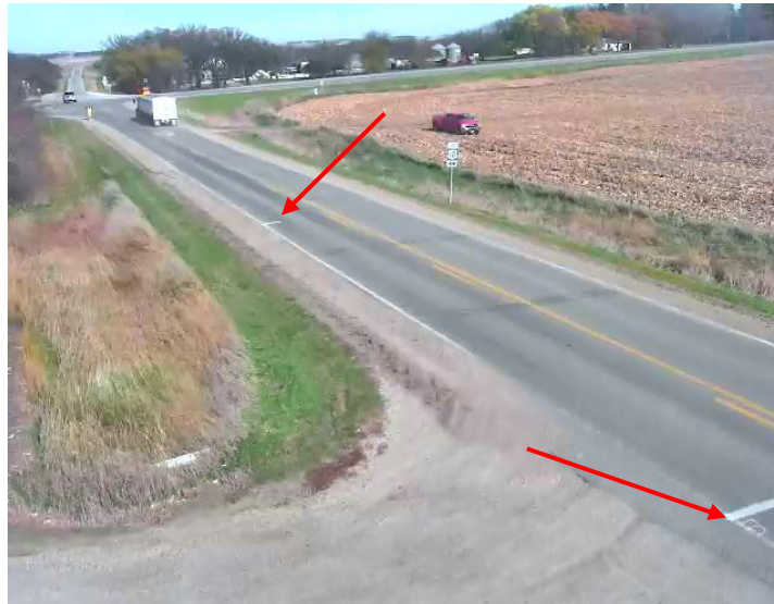
Figure 4-3. White lines marked in the field
