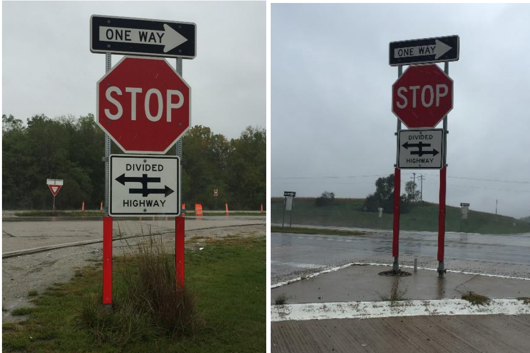
Figure 3-2. Reflective strip installation at four-lane divided highways
