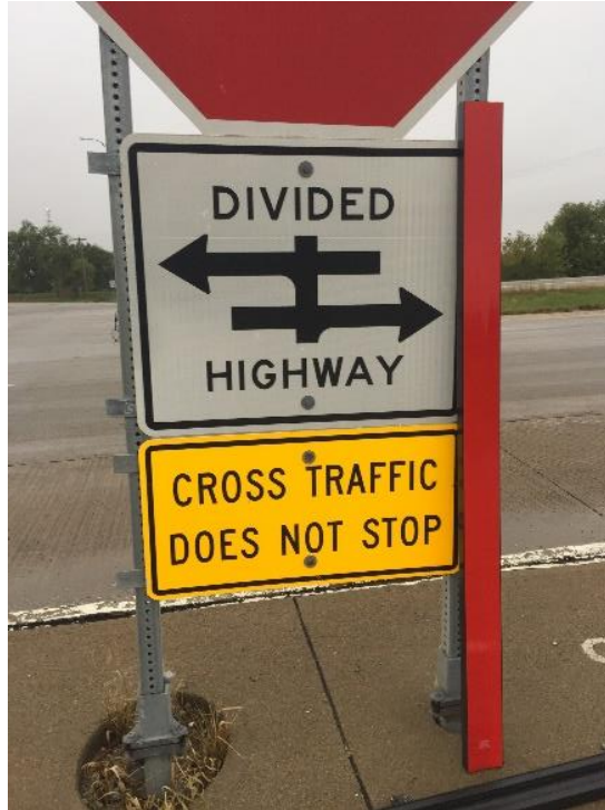
Figure 3-6. Installation not possible due to sign and spacing constraints
