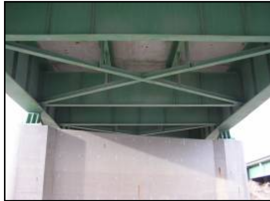
b. Girders, stringers, floor beams, and stiffeners c. Cross bracing
