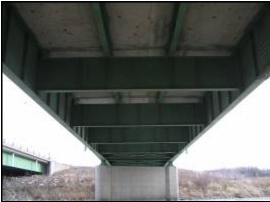
b. Girders, stringers, floor beams, and stiffeners c. Cross bracing
