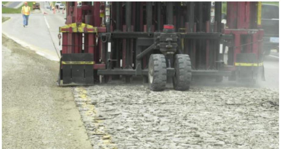
*Rubblization using a multiple-head breaker*
