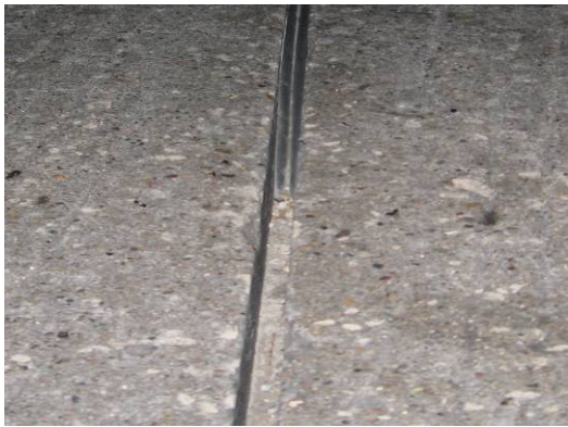
(b) Joint sealing damage of transverse joint at slab #3
