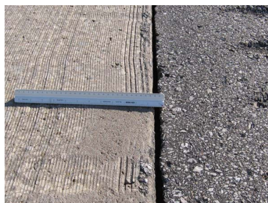
(b) Lane to shoulder separation at slab #9
