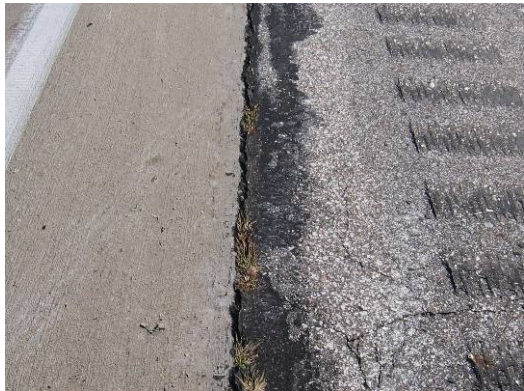
(a) Lane to shoulder separation at slab #2
