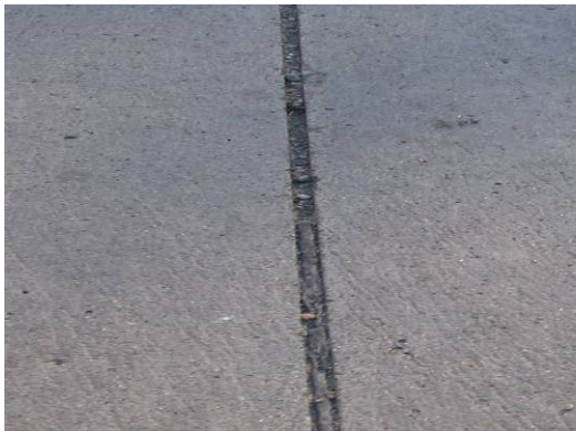
(b) Joint sealing damage of longitudinal joint at slab #6
