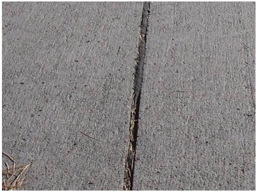
(c) Joint sealing damage of longitudinal joint at slab #8
