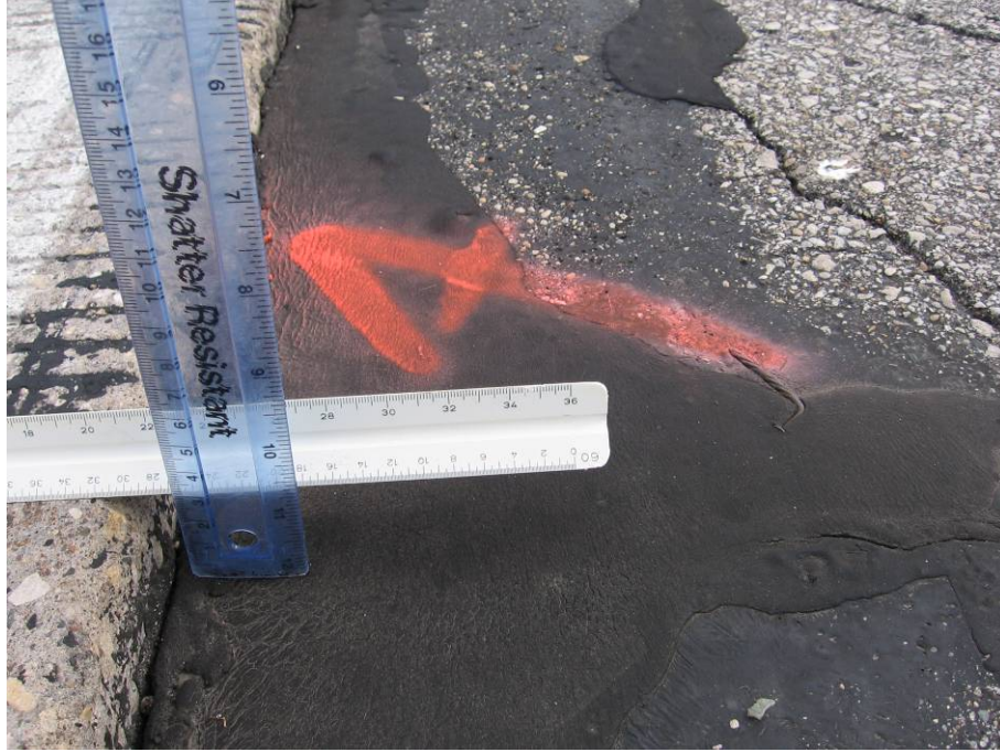
Figure 24. Lane to shoulder drop off on I-35(N) in Hamilton County (Mile Post No. 131.40–131.45)—RPCC subbase section
