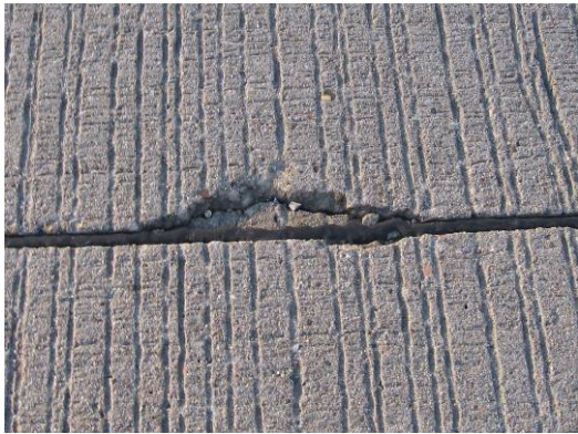
(c) Spalling of longitudinal joint at slab #10
