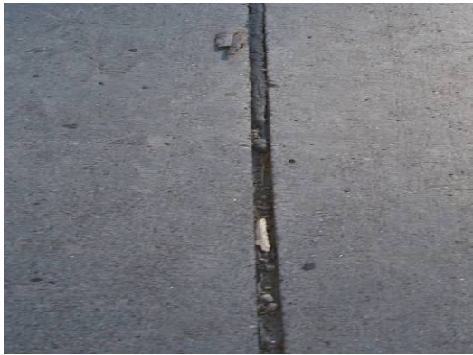
(d) Joint sealing damage of transverse joint at slab #12
