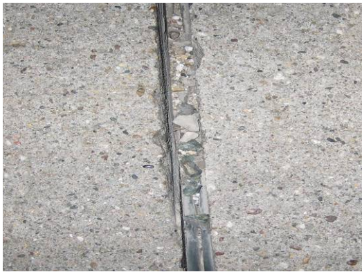
(b) Joint sealing damage of transverse joint at slab #4
