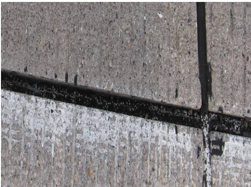
(b) Joint sealing damage of longitudinal joint at slab #5
