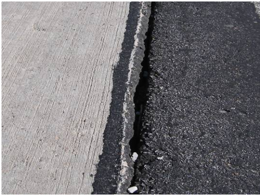
(a) Lane to shoulder separation at slab #1
