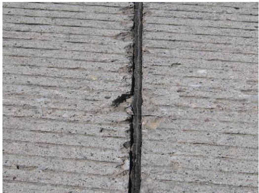
(c) Spalling of transverse joint at slab #14
