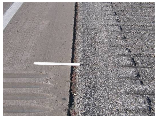
(c) Lane to shoulder separation at slab #17
