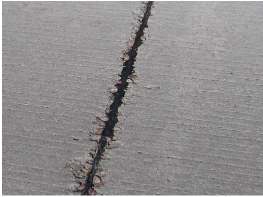
(b) Spalling of transverse joint at slab #5
