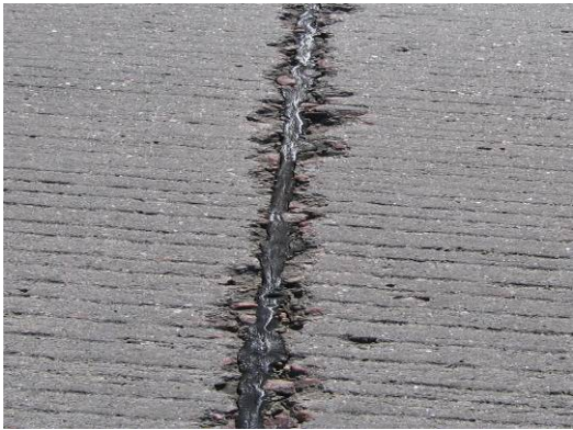
(c) Spalling of transverse joint at slab #7
