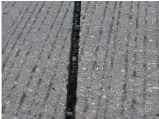
(a) Joint sealing damage of transverse joint at slab #1
