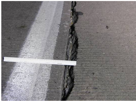
(a) Lane to shoulder separation at slab #1
