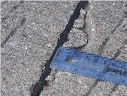
(a) Spalling of transverse joint at slab #4
