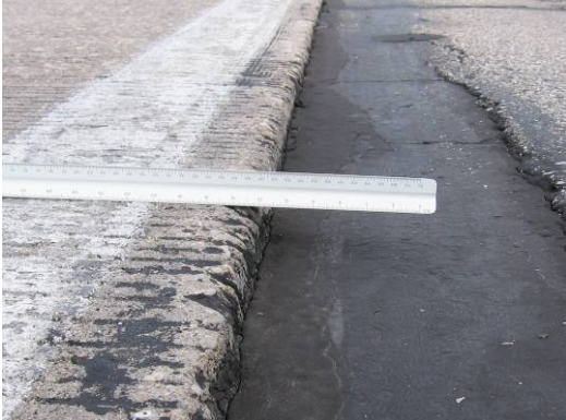
(a) Lane to shoulder drop-off at slab #1
