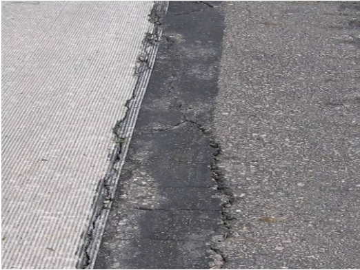
(c) Lane to shoulder separation at slab #15
