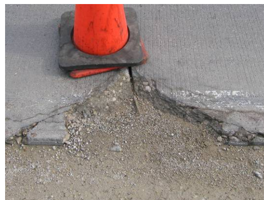
(b) Corner break at slab #12 and #13
