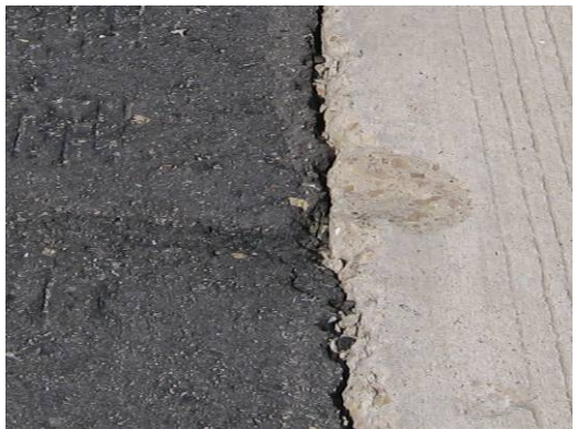
(b) Lane to shoulder separation at slab #5
