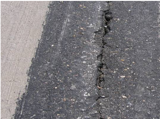
(c) Lane to shoulder separation at slab #11
