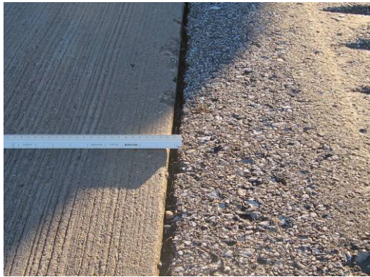
(a) Lane to shoulder separation at slab #3
