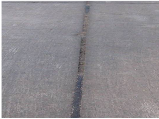
(c) Joint sealing damage of longitudinal joint at slab #2
