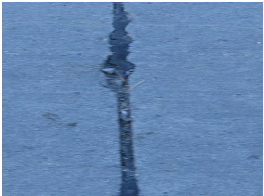
(a) Joint sealing damage of transverse joint at slab #3
