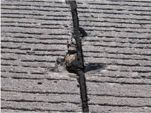
(c) Spalling of transverse joint at slab #9
