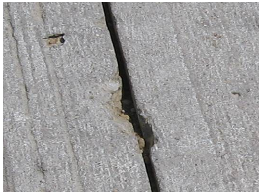
(c) Spalling of longitudinal joint at slab #15
