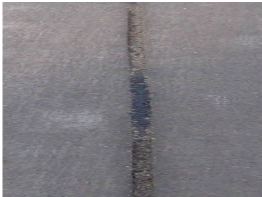
(a) Joint sealing damage of longitudinal joint at slab #1
