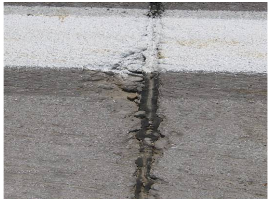
(b) Spalling of transverse joint at slab #12
