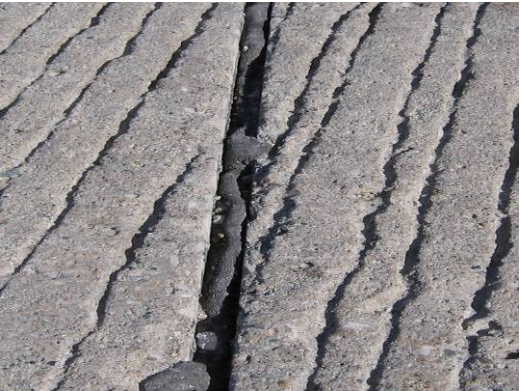
(b) Joint sealing damage of transverse joint at slab #6
