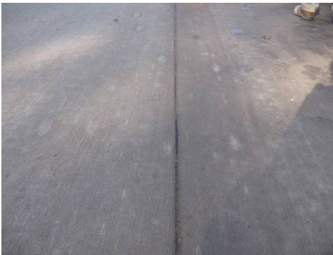
(a) Joint sealing damage of longitudinal joint at slab #1
