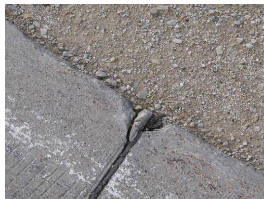
(c) Spalling of transverse joint at slab #14
