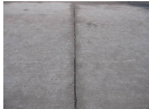
(d) Joint sealing damage of transverse joint at slab #2
