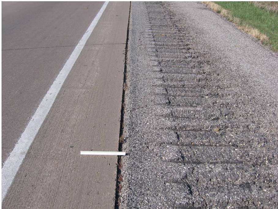
Figure 23. Lane to shoulder separation on I-80 (W) in Cedar County (Mile Post No. 269.30–269.40)—RPCC subbase section
