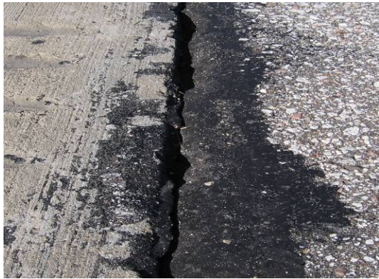
(c) Lane to shoulder separation at slab #15
