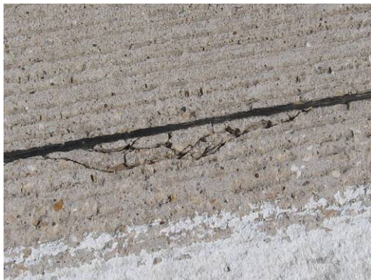
(a) Spalling of longitudinal joint at slab #4
