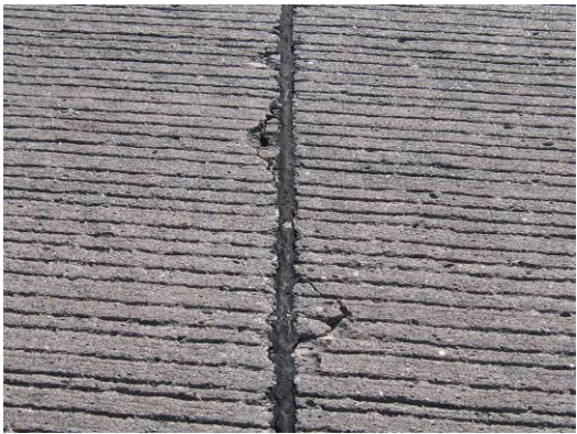
(b) Spalling of transverse joint at slab #5
