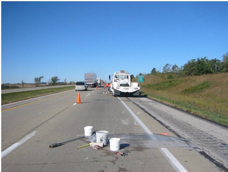
Figure 8. Coring and preparation for field tests
