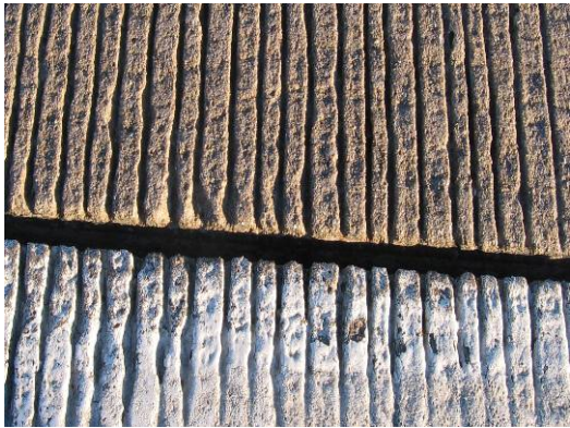
(b) Joint sealing damage of longitudinal joint at slab #4
