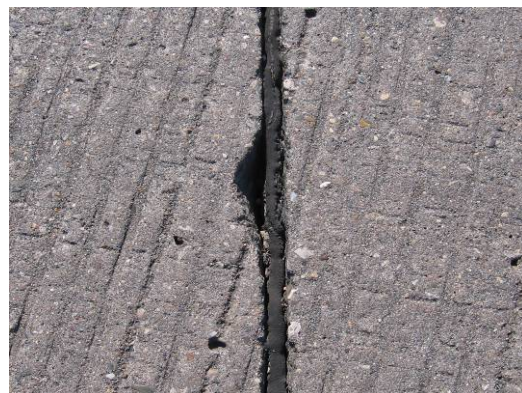
(b) Spalling of transverse joint at slab #12
