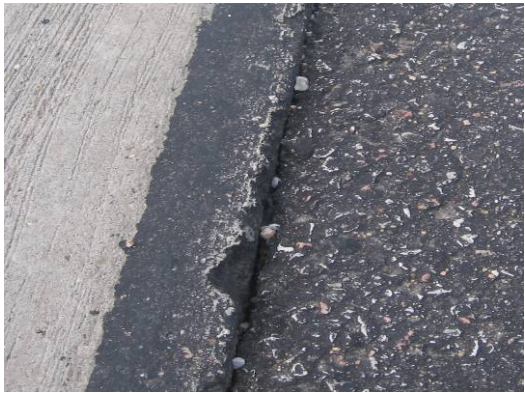
(a) Lane to shoulder separation at slab #2
