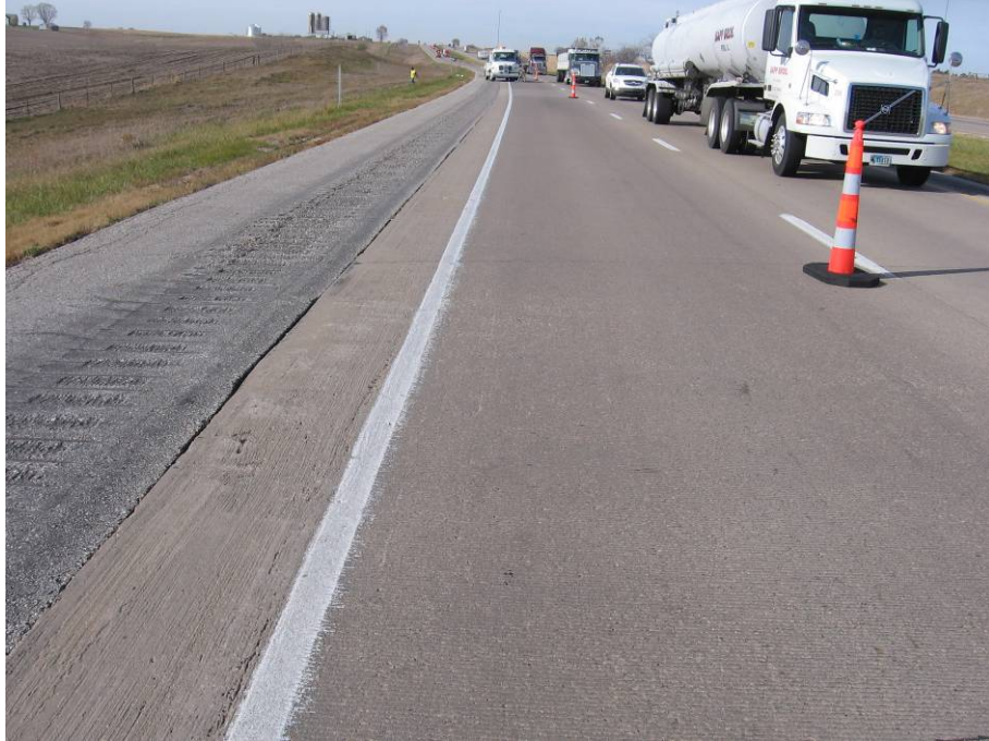
Figure 22. Picture of I-80 (E) pavement section in Cedar County (Mile Post No. 276.60–276.70)—RPCC subbase section
