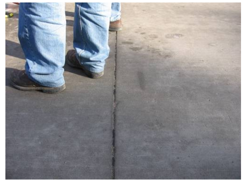
(b) Joint sealing damage of transverse joint at slab #1
