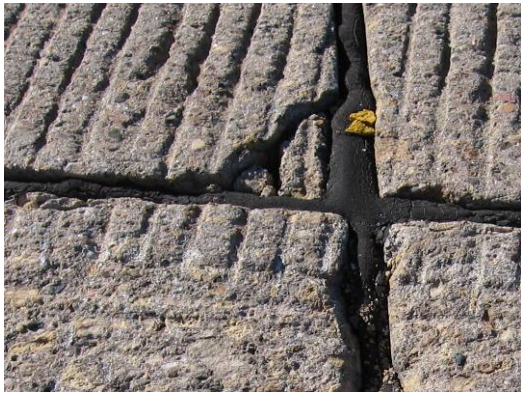
(b) Spalling of transverse joint at slab #5
