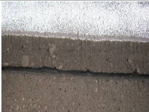
(a) Spalling of longitudinal joint at slab #1
