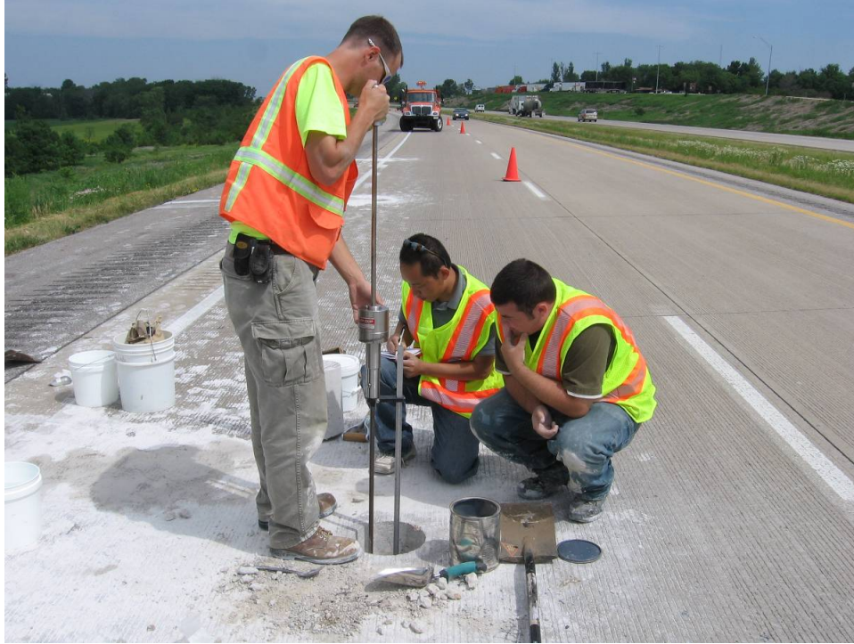
Figure 10. Dynamic cone penetrometer (DCP) test
