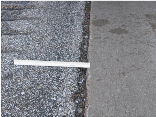
(b) Lane to shoulder separation at slab #5
