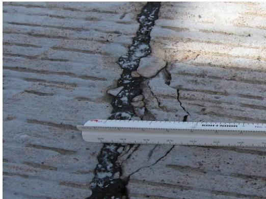
(c) Spalling of Transverse joint at slab #6
