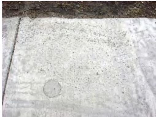
**Figure 6–39. Scaling of SFSCC at South 4th Street in March 2009**
