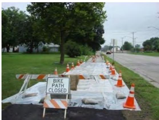
**Figure 6–19. Curing of concrete, South 4th Street**
