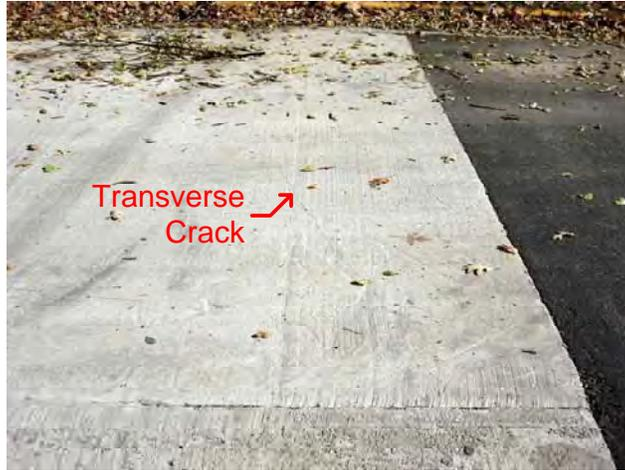
**Figure 6–48. Transverse crack at North Riverside Drive SFSCC pavement located at NR-M3-A mix as of October 2008**
