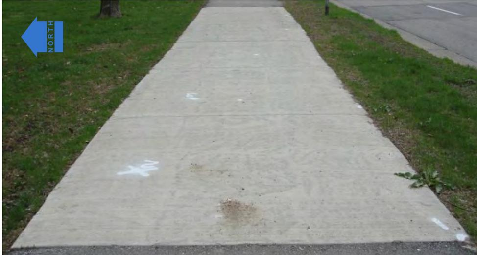
**Figure 6–40. Condition of SFSCC pavement at South 4th Street on April 2011**
