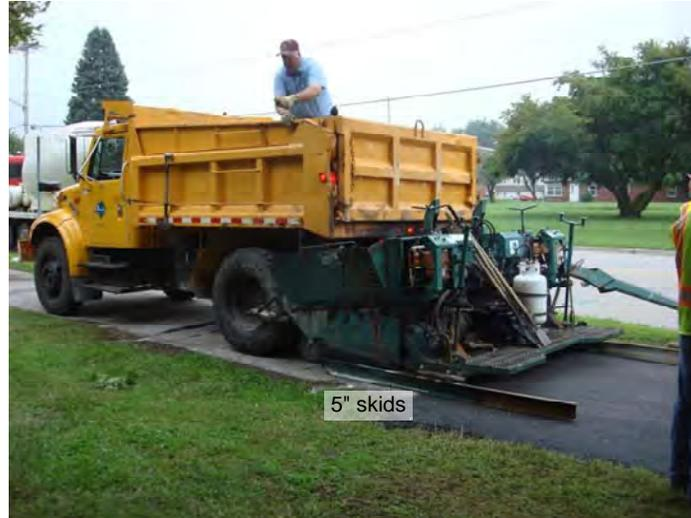
**Figure 6–9. Modified asphalt paver for slip-form paving**
