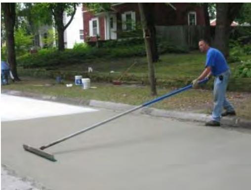
**Figure 6-30. Brooming for surface texture, North Riverside Drive**
