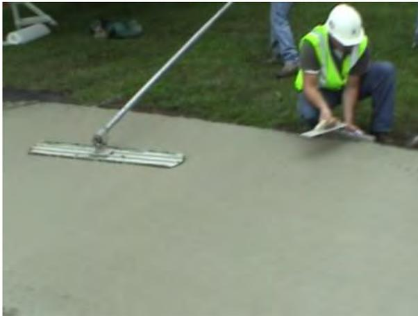
**Figure 6–16. Finishing of pavement, South 4th Street**
