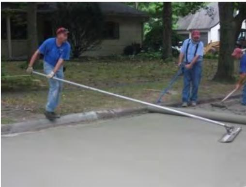
**Figure 6-29. Finishing of pavement, North Riverside Drive**
