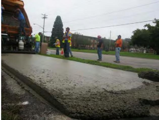
**Figure 6–13. S4TH-M1 slab before finishing**
