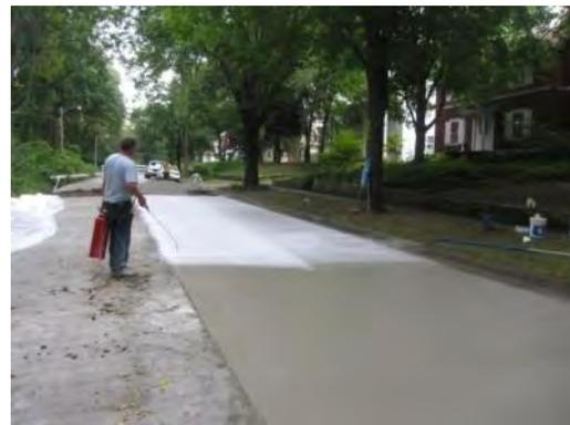
**Figure 6-31. Application of curing compound, North Riverside Drive**
