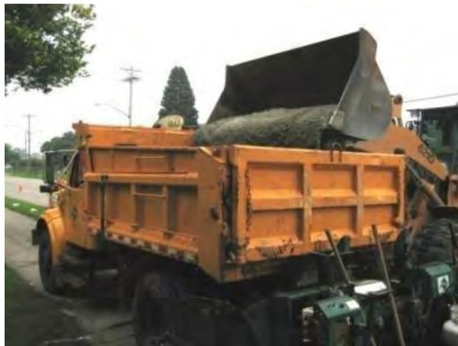
**Figure 6–12. Concrete was first transported into a dump truck and then loaded into the paver**
