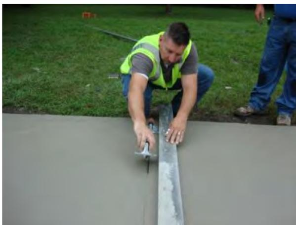
**Figure 6–17. Cutting of joint, South 4th Street**
