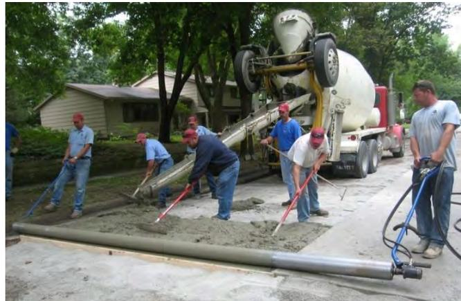
**Figure 6–24. Roller screed for leveling of poured concrete**
