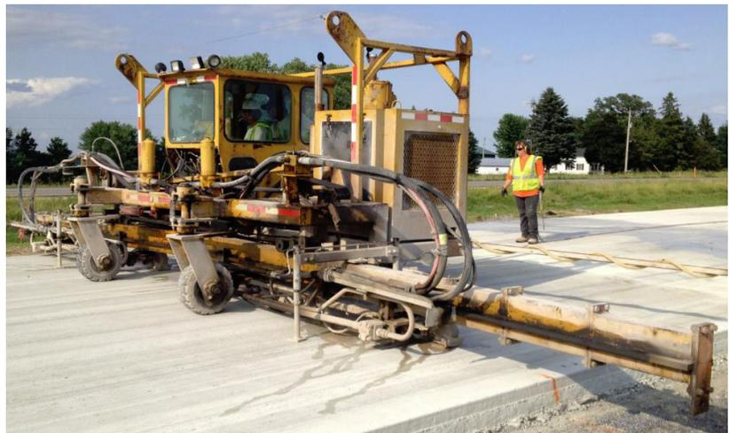
*Non-typical conventional gang-saw machine used at one site*
