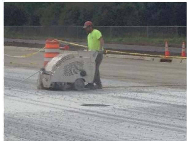
*Typical early entry saw-cutting process*
