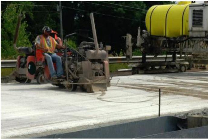
*Typical conventional saw-cutting process*
