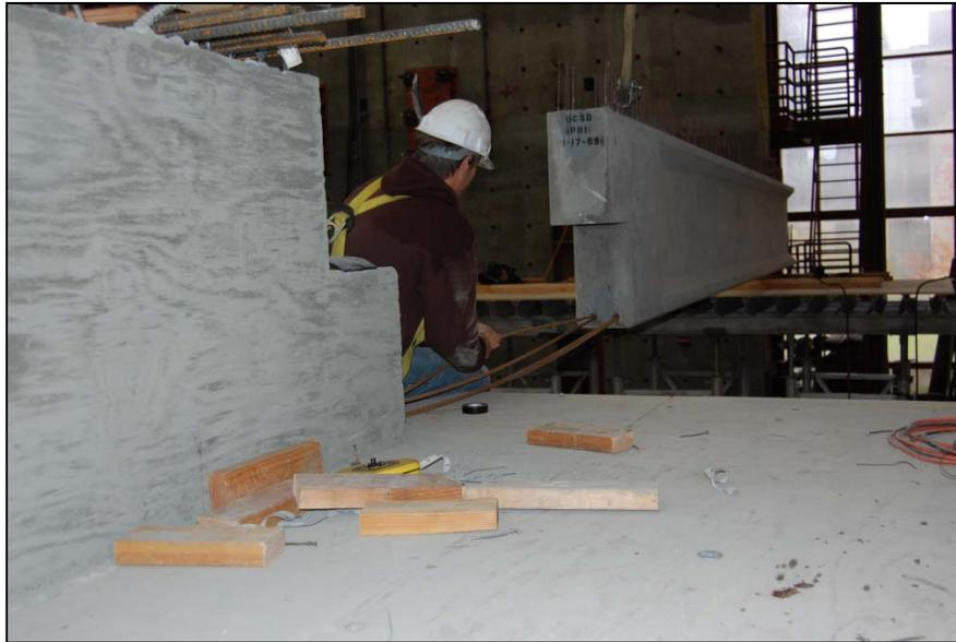
Figure 5.11: Pushing the Strands through the Girder
