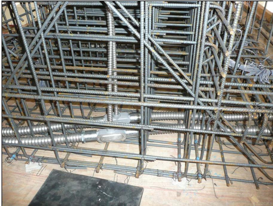
Figure 5.9: Routing of Bent Cap Ducts
