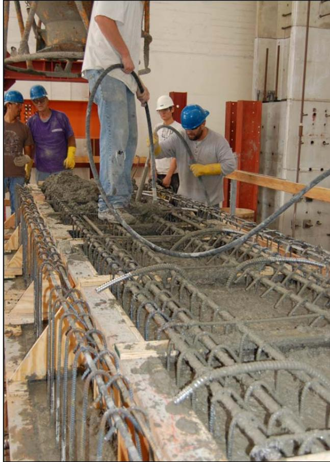
Figure 5.8: Casting of the Bent Cap
