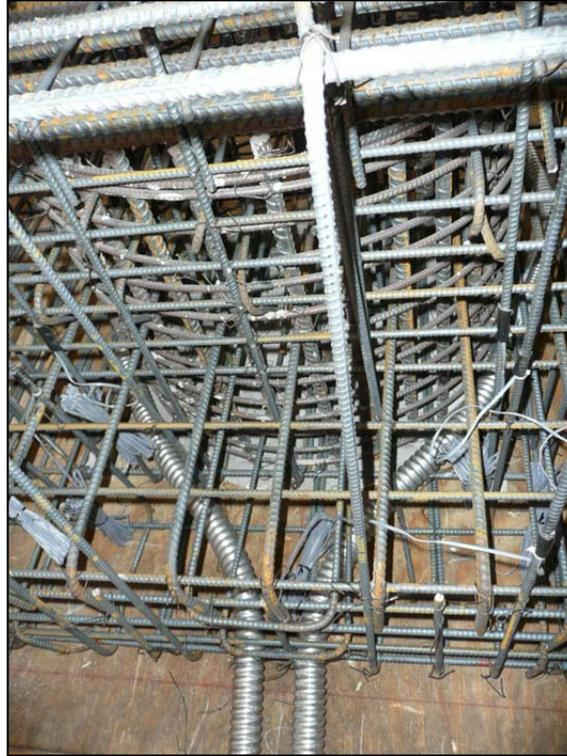
Figure 5.10: Placement of Ducts in the Bent Cap around the Column
