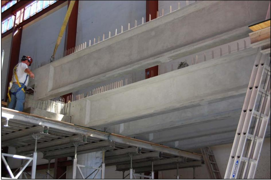
Figure 5.5: Installation of Southern Girders
