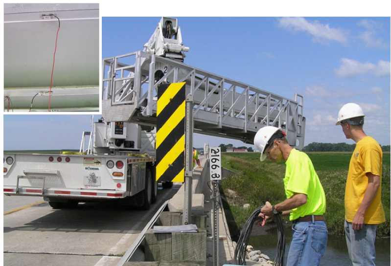
US-18 bridge east of Hartley, Iowa, being instrumented
